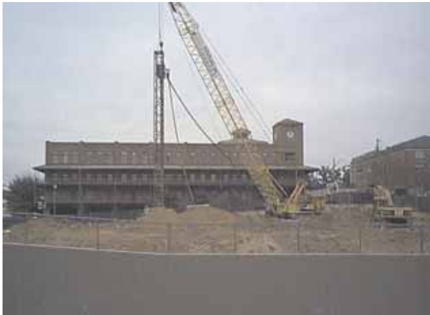
Construction of the Challenger Center/IMAX
