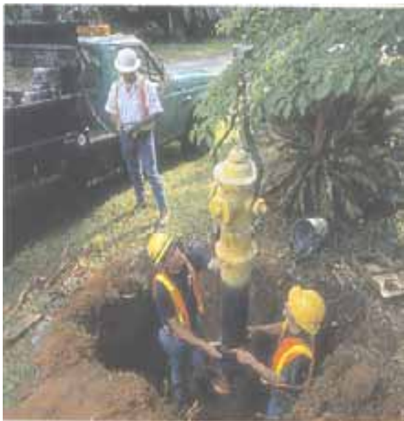
Water Utility Crew Working on Fire Hydrant
