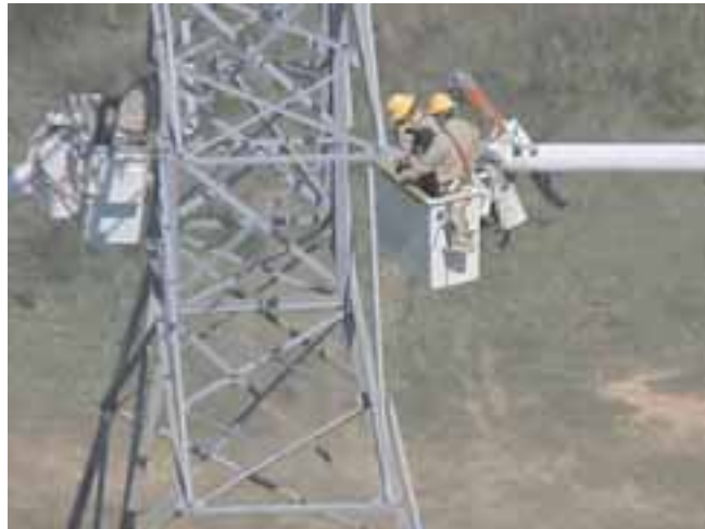
T&D Crew at Work on a Transmission Tower
