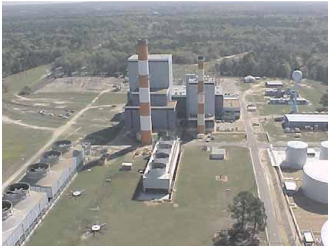
Arvah B. Hopkins Generating Station
