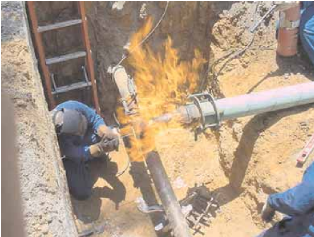
Gas Utility Workers Repairing a Gas Main
